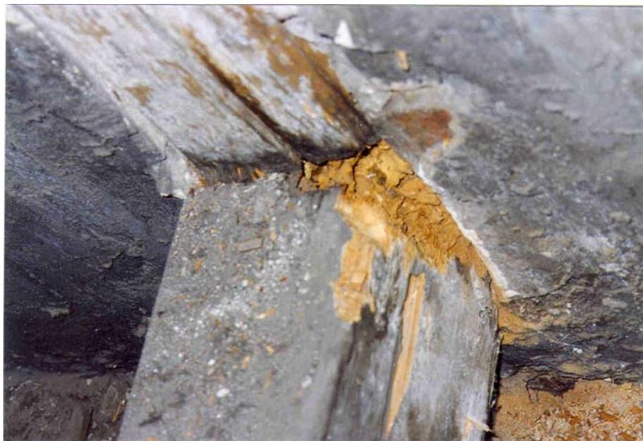
*Figure 6. Beam Head Failure*
