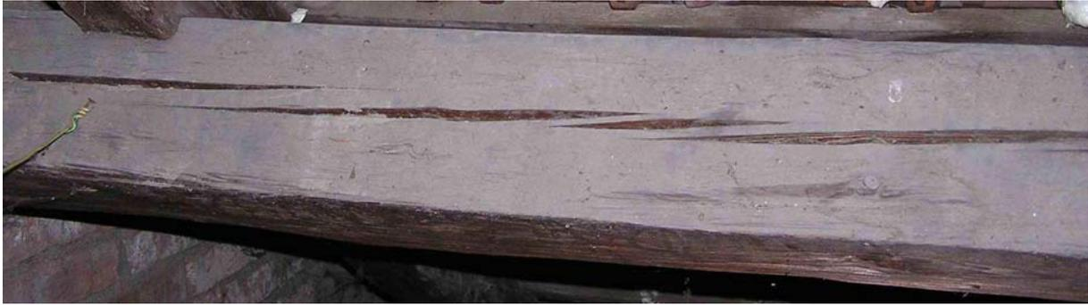
*Figure 3. Shrink Crack in a Roof Element*
