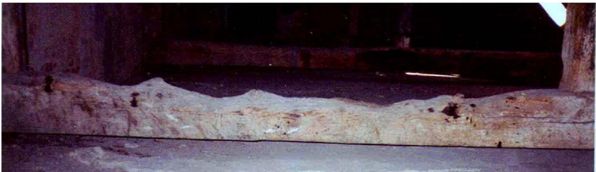
*Figure 2. Beam Mechanical Damage (cross-sections reduction due to wood chopping)*
