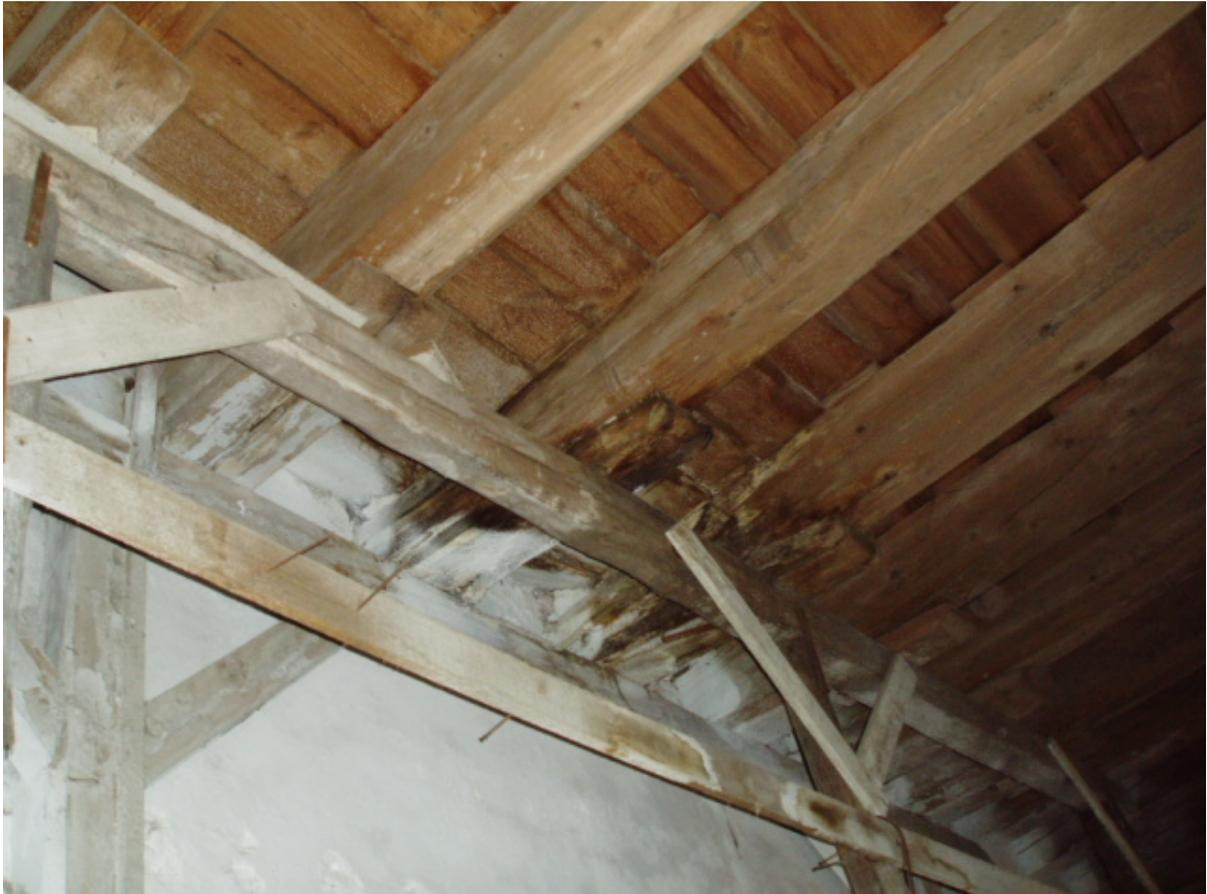
*Figure 1. Roof In-Leak*
