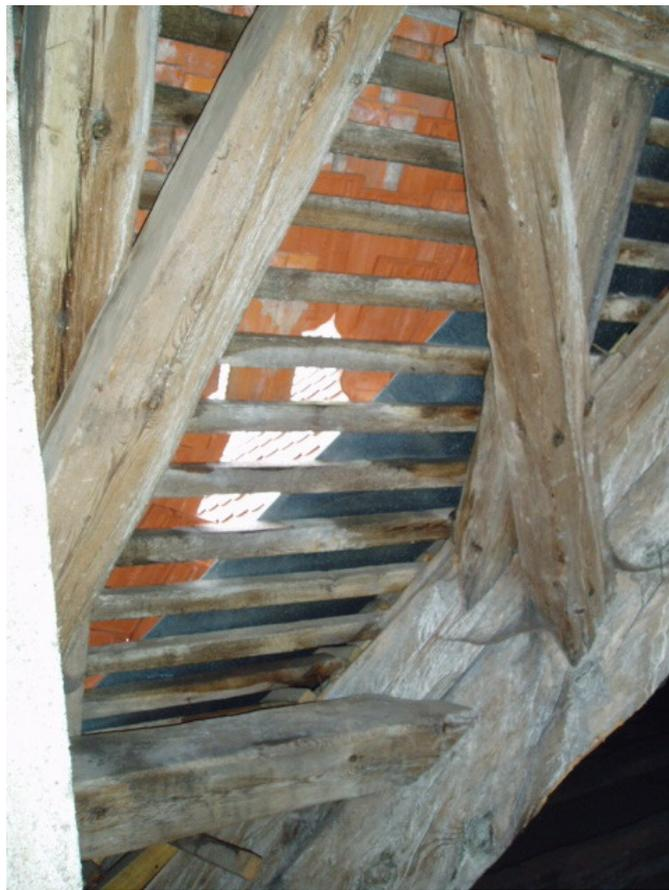
*Figure 4. Knags in a Roof Beam*
