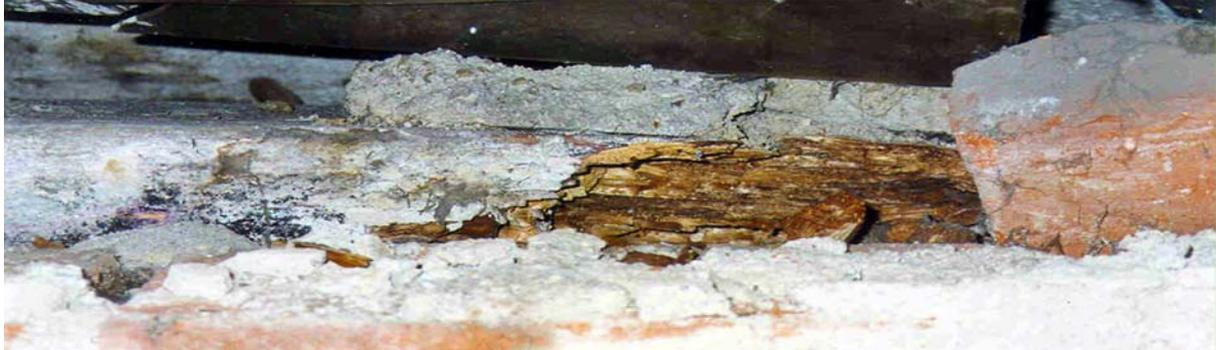
*Figure 5. Roof Failure Due to House Fungus Attack*
