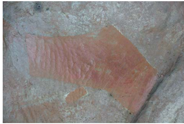
Fig.6-7 A Monument's particular without and with a coat of pigments mixed with solvents.
