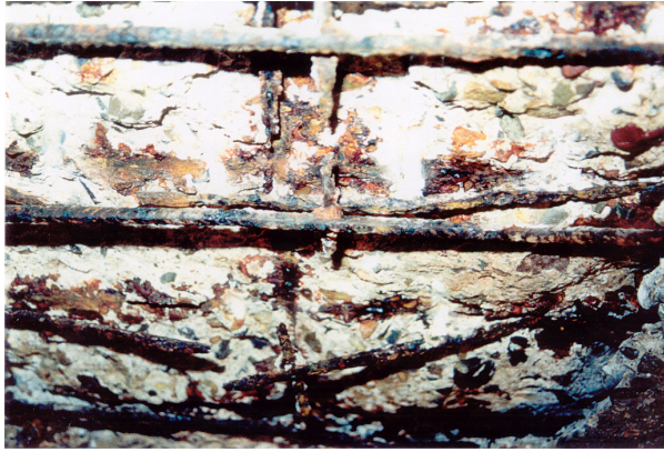
(a) Reinforcement steel with concentrated loss of section caused by pitting corrosion from de-icing salts. (b) Concrete corrosion with deterioration of the surface near concrete caused by sewage water in a sewage treatment plant.
