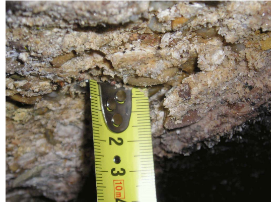
(a) Reinforcement steel with concentrated loss of section caused by pitting corrosion from de-icing salts. (b) Concrete corrosion with deterioration of the surface near concrete caused by sewage water in a sewage treatment plant.
