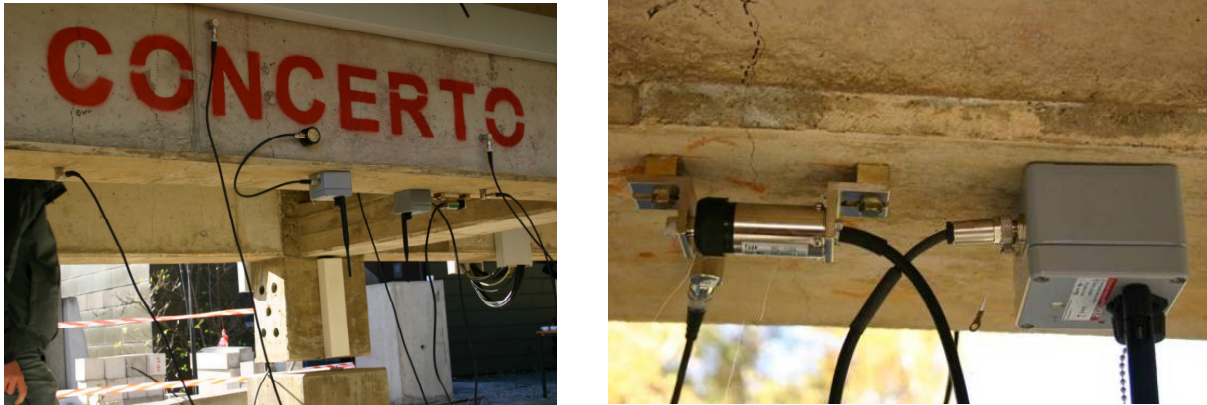
Figure 4. Bridge equipped with wireless AE sensors (left) and with wireless displacement sensors (right)
