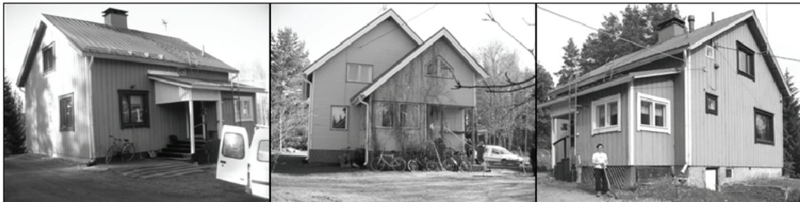
Figure 1. The studied houses represent the typical single-family houses built in the 1940's and 1950's. Their air tightness is relatively low according to recent studies.
