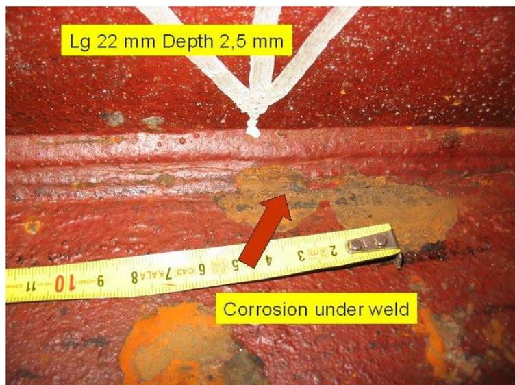
Figure 11. Localised corrosion under weld toe
