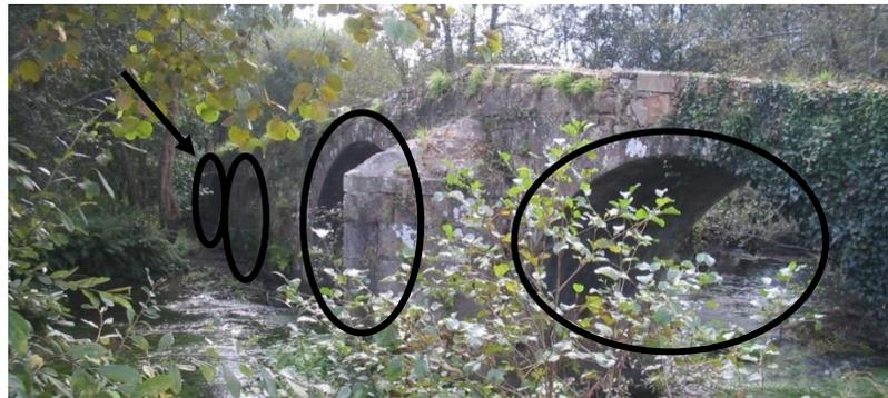
**Fig.2.** Side view of the Lubiáns Bridge, with its four arches highlighted by black circles. The arrow points the arch subject of deeper study due to a previous detection of moisture in it.
