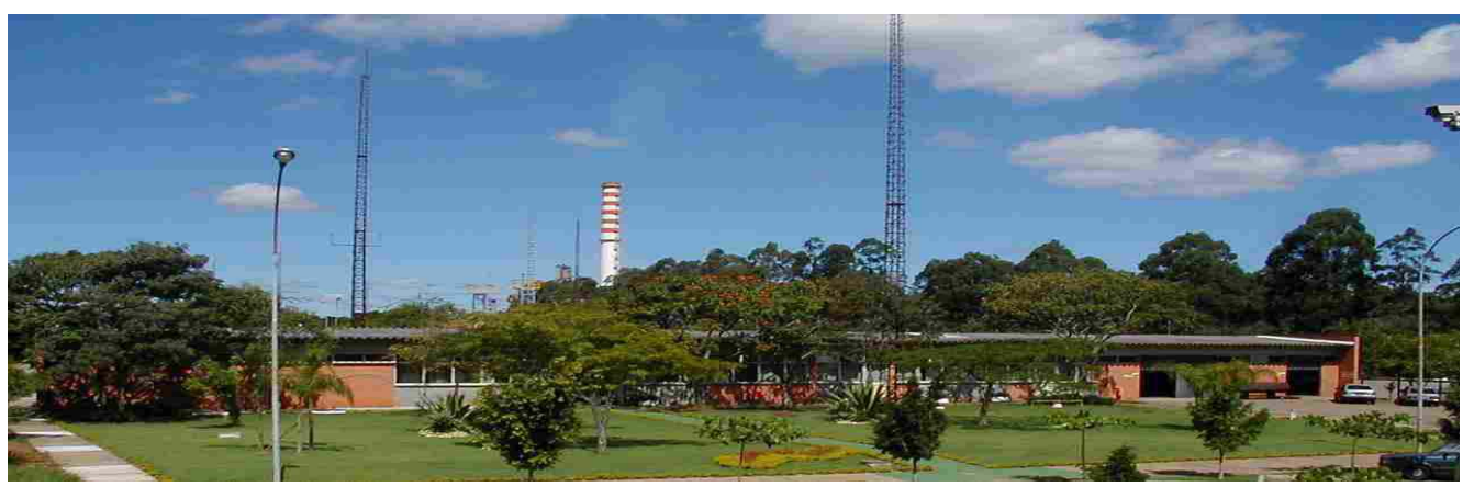
PETROBRAS/SEQUI Facilities - Examination Center - São José dos Campos, Brazil
