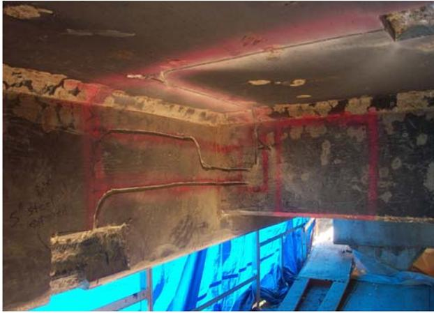
Figure 8. Installation Area for Strain Sensors
