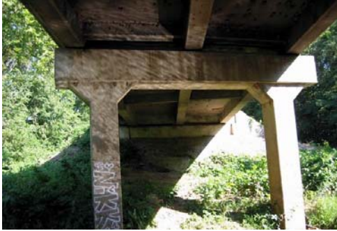
RC Bent, Girders and Slab
