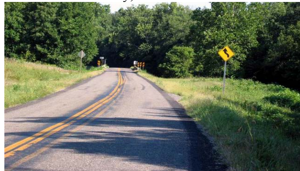
Approach to the Bridge
