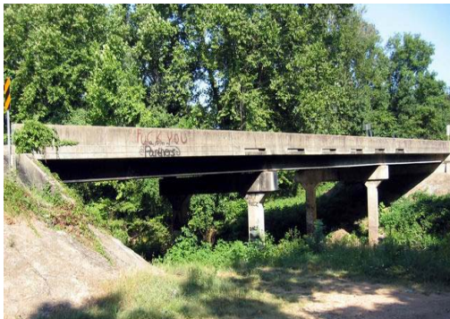
Side View of the Bridge
