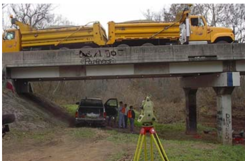
a) Surveying Equipment.
