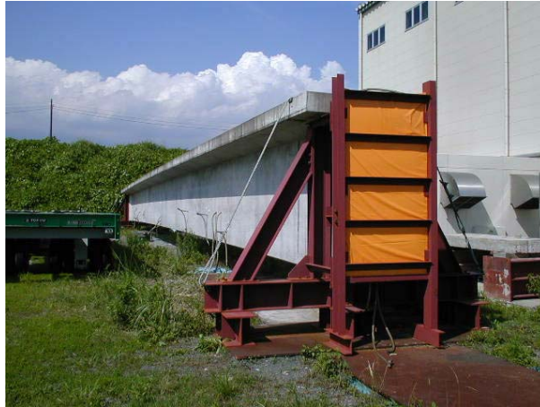
Photo 1 Actual-size pre-stressed girder
