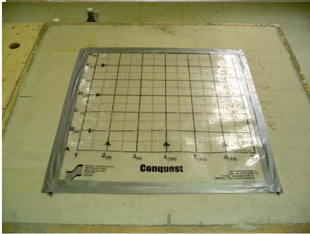
Figure 1: Test pad construction prior to concrete pour.
