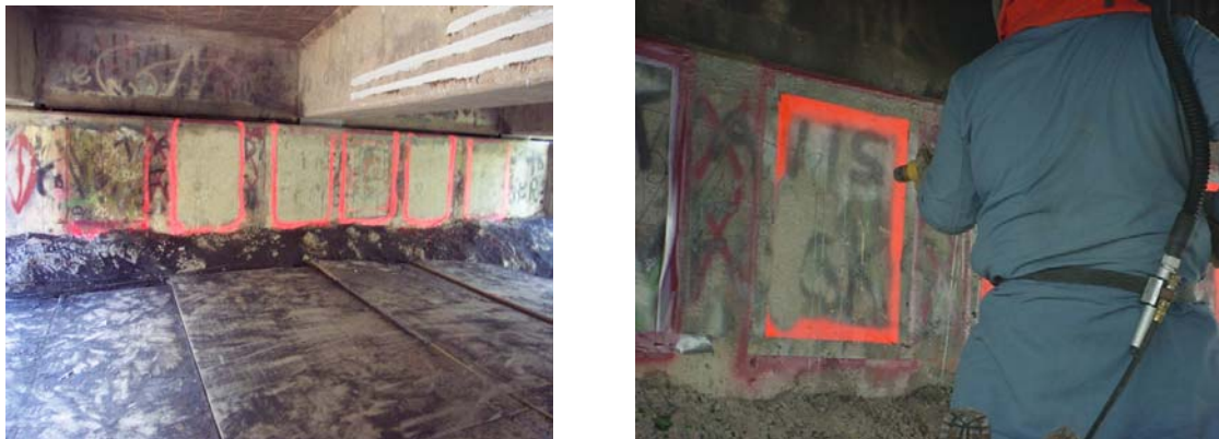
Figure 2. Surface Preparation on Abutment
