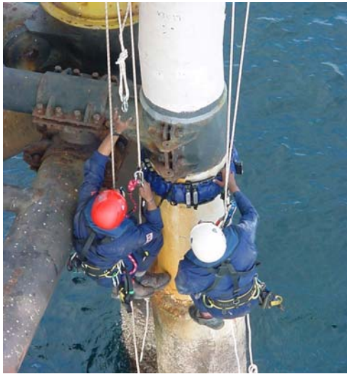
Fig 2. Flexible transducer ring deployed offshore.
