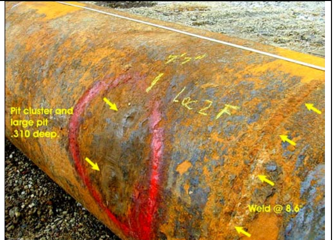
Figure 3. Large isolated pits in front of a weld. See Figure 6 showing signal response from this area – 7 to 9 feet.
