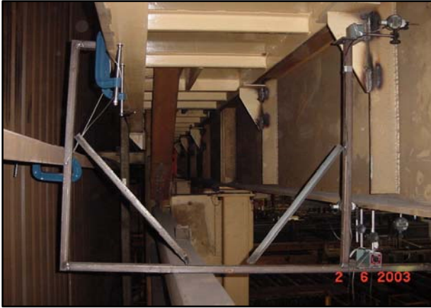
Picture No 2: Set-up for digital indicators installation
