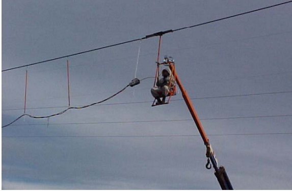
Figure 7 : Test arrangement on a 230 kV energized line
