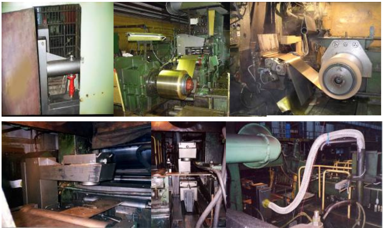
Fig.2. RIT10 X-ray Thickness Gages at the Rolling Shop
