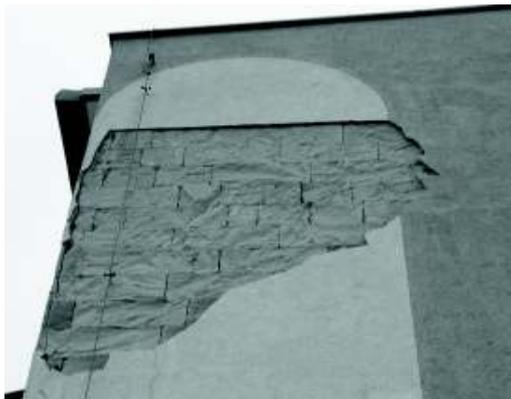
Fig. 2. Cement-lime plaster coming off gas concrete wall in area of few m<sup>2</sup>.
