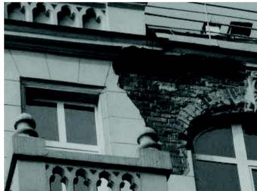
Fig. 3. Cement-lime plaster and mascarons falling off ceramic brick wall in area of 1.5 m<sup>2</sup>.
