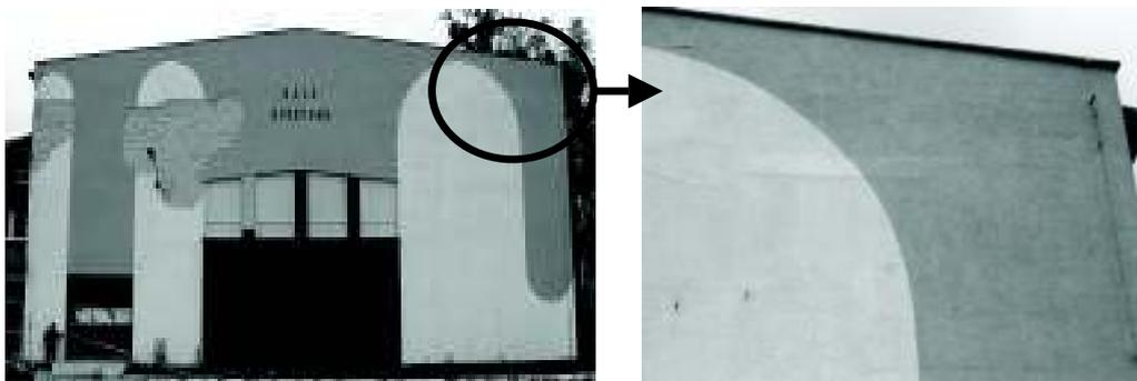
Fig. 1. View of part of industrial building (left) and close-up of plaster. Clearly visible network of cracks (right).
