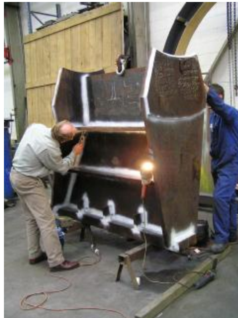
Photo 3 The new arm under construction.
