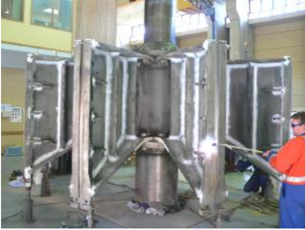
Photo 4 NDT and weld repairs of the rotor
