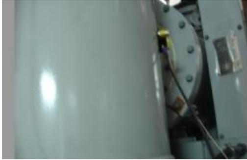
Figure 4 : The AE sensor measurement position.
