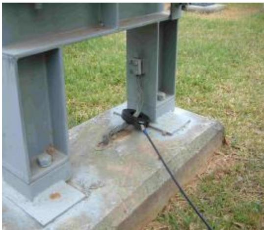
Figure 2: *The on-line PD measurement using a HF-CT.*
