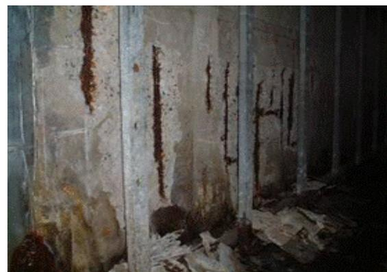
Fig.3 Cable tunnel degradation conditions construction
