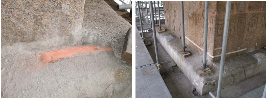
Fig. 32,33. Metallic brackets on the corner of obelisk
