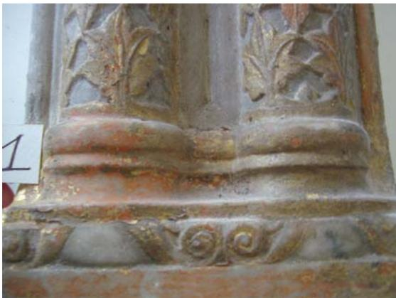
Figure 2. Basement of the column on the left side of the left panel. Missing gilding layer showed the behind red preparation layer.
