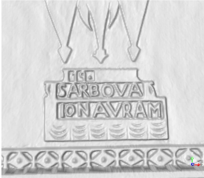
A detail from the upper part of the facade, mesh visualization, medium resolution: 1 mm
