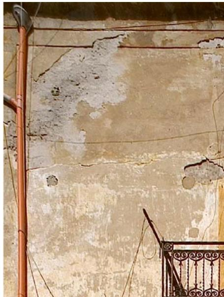
*Pict.2 Detail of the current status of the facade. IRT was made on 2007/09/17 at 20.30 p.m. after sunset in the direct cooling down phase temperature +31°C, relative humidity 34%*
