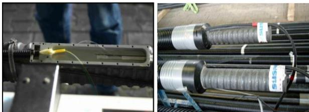
Figure 7: Splice box (left) and cable protection at the anchor's pile head (right).
