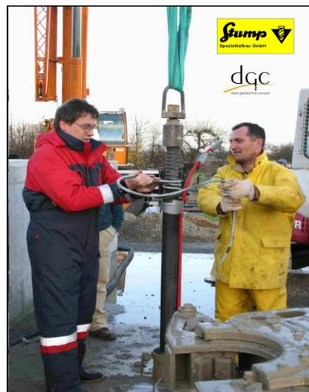
Figure 8: Introduction of the micro pile into the bore hole.
