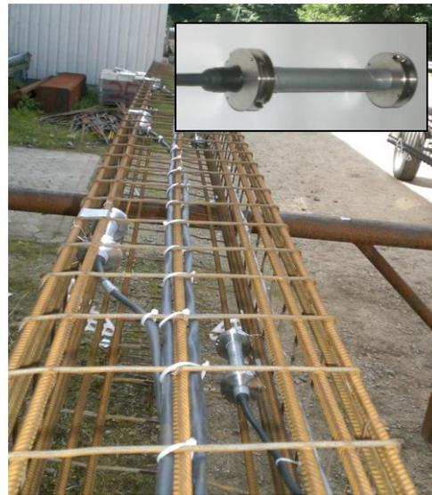
Figure 5: Sensors fixed at the cage of reinforcement for a 19 m long concrete pile (above right: sensor body)
