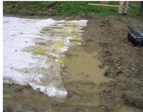
Figure 12: Sensor-based geotextile mat during the installation on a construction site of a gravity dam in Solina/Poland (Textile: STFI e.V. Chemnitz).
