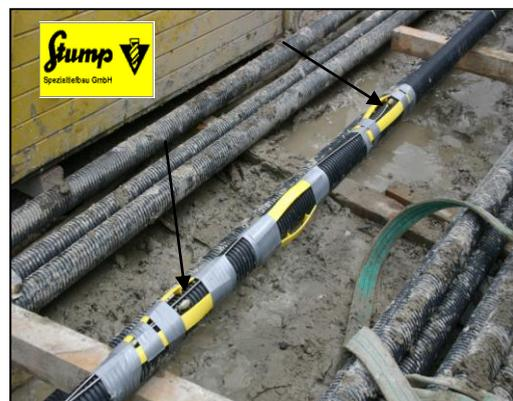
Figure 18: Prefabricated anchors with fixed pH sensors (arrows). Photo: BAM
