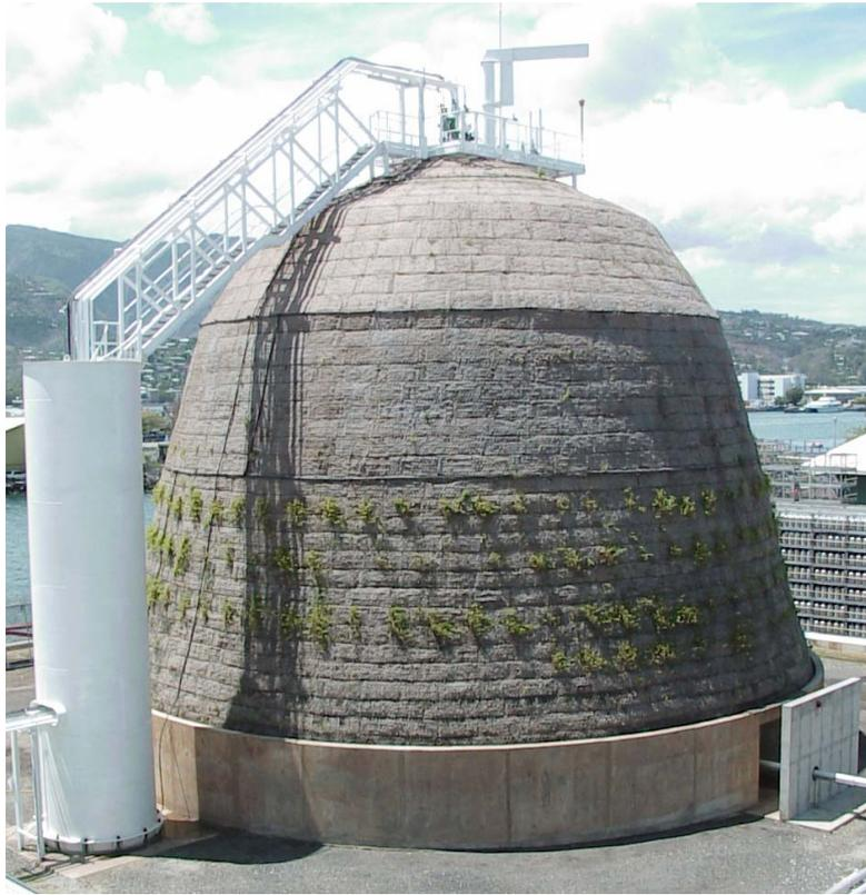
**Figure 5:** Substitution of the hydraulic proof test of a spherical storage tank by a pneumatic test monitored by acoustic emission
