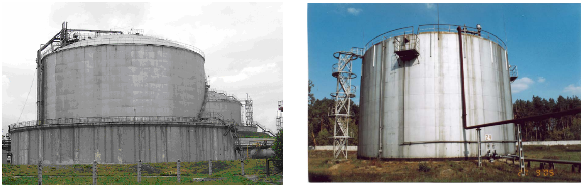
Fig. 1. General view of welded tanks for liquid ammonia storage.
