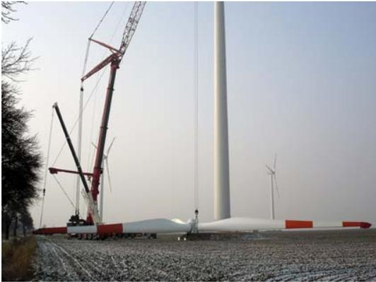
Fig. 19: Removing the three blades from the generator and placing it on the ground.
