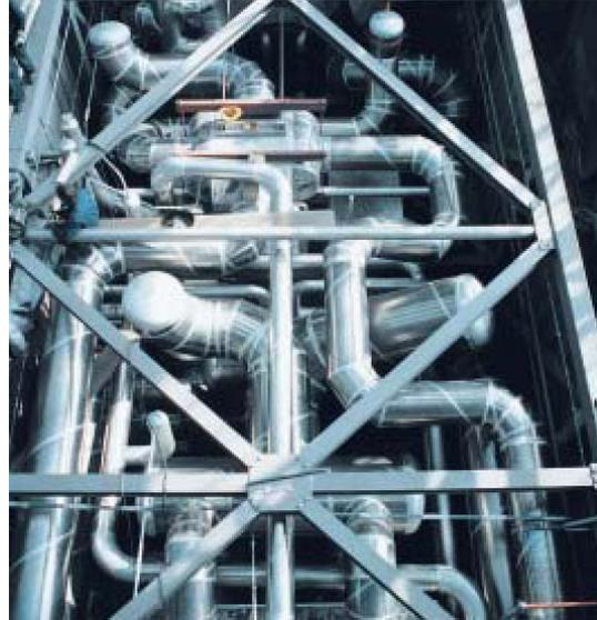
Figure 2: Typical structure of the piping and equipment inside a cold box.
