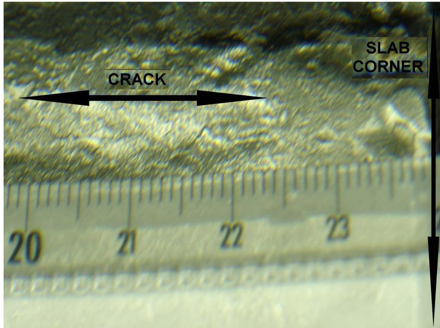
**Figure 11:** Crack aspect under magnifying glass. The arrow shows the slab corner.
