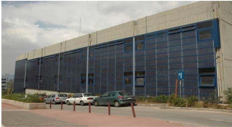
Figure 2 : Buildings façade with the first six PV arrays
