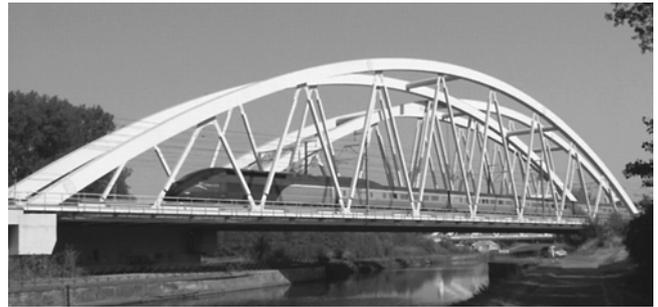
Figure 1. Tied arch bridges with orthotropic plated deck at Halle (Belgium)
