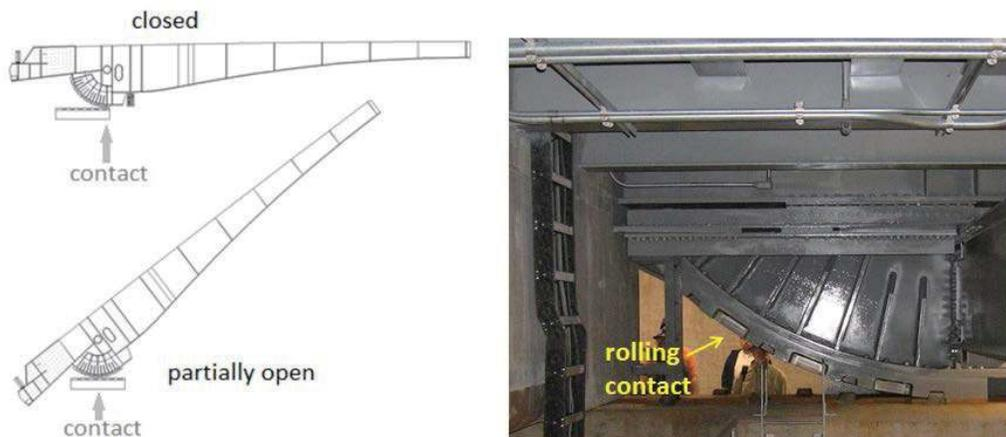
Figure 4: Sketch of bascule bridge leaf and photograph of bascule girder heel showing moving contact areas
