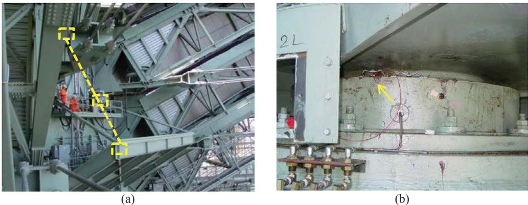
Figure 2: (a) Annotated photograph showing one side of tree-like structure supporting the five roof panel pivot bearings; (b) close-up of typical roof panel bearing showing location of AE transducer
