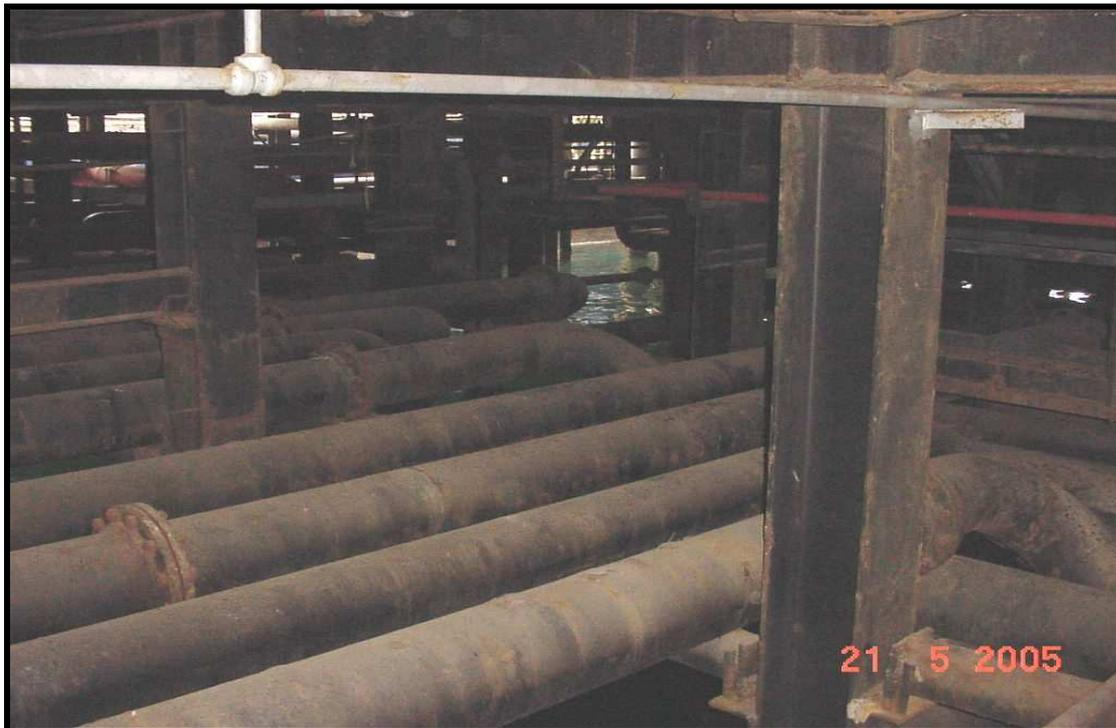
*Photo 1: Layout of Sea Lines under Wharf's deck.*
