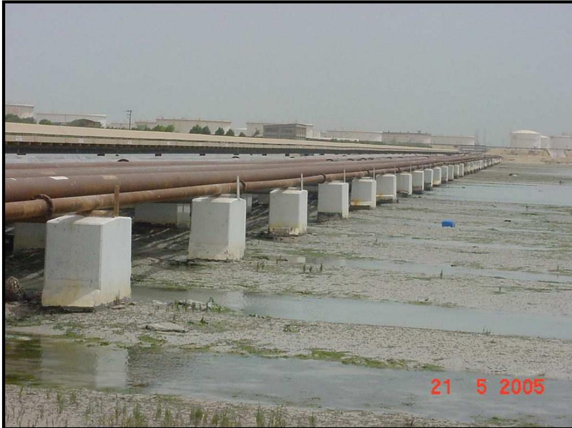
*Photo 5: Supports of transfer lines at Wet Gap.*
