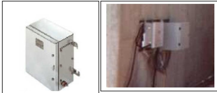
**Figure 3: EExe packaging of 16 channel node with barriers for use in hazardous environments with I.S. sensors (left), right is field packaging for non hazardous environment (small box).**
