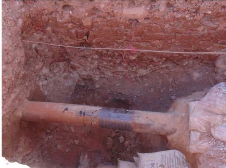
Figure 7. Exposed section of 8 inch pipe. A small portion of coating was removed (0.5m length) in order to couple the ring onto the pipe.
