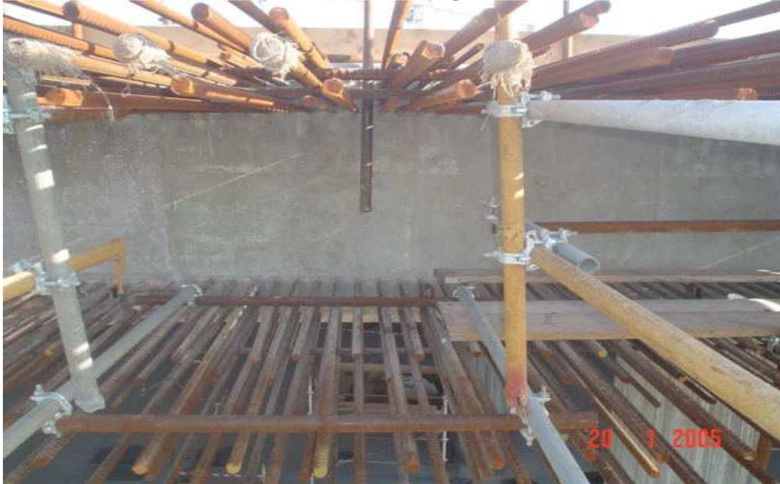
**Figure 14: A picture taken of the side of the exposed Slab which clearly displays a sample of the reinforcement configuration. The slabe is 1.5 meters thick.**
