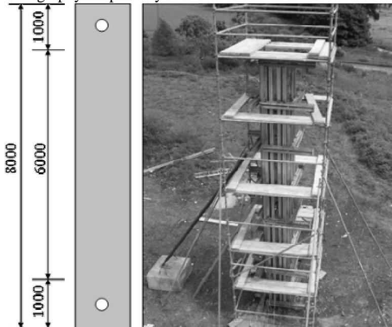
**Figure 1** Locations of the cores (base and top) on 8.0 m column, (units are in mm),
