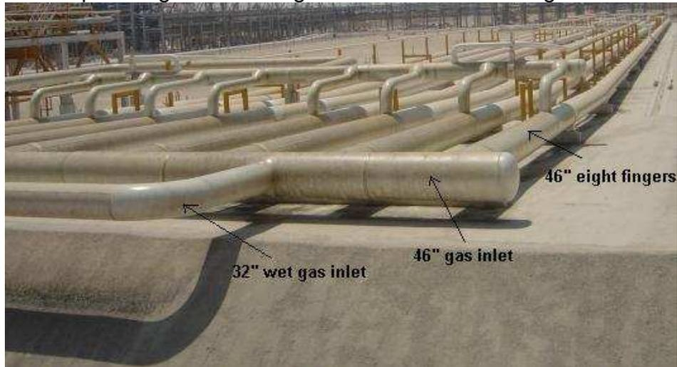
Figure 1: Slug Catcher – view from inlet side
