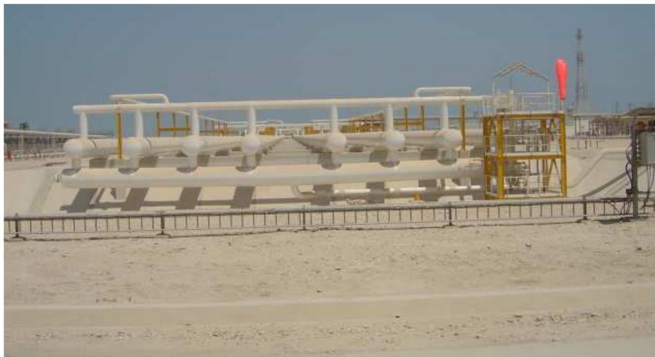
Figure 2: Slug Catcher – view from liquid header side
