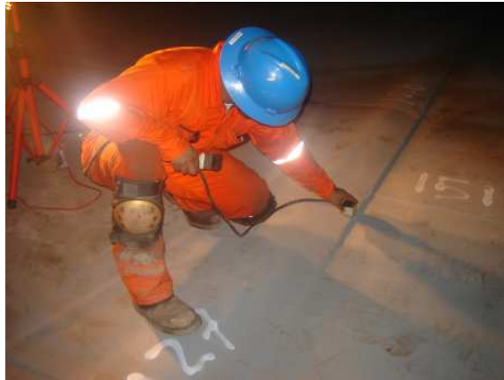
Fig 12. Inspection of floor weld with standard weld probe
