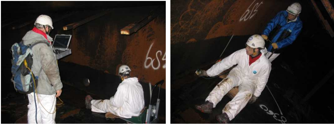
Figure 6. High speed inspection of wall to floor weld
