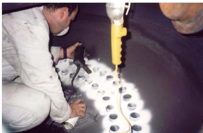
Fig. 5: Examination of tube-to-drum joints using magnetic particles.
