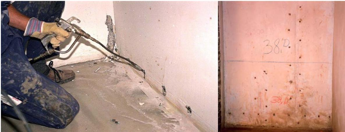
Fig. 3: Crack repair by injection and a photo of repair position.
