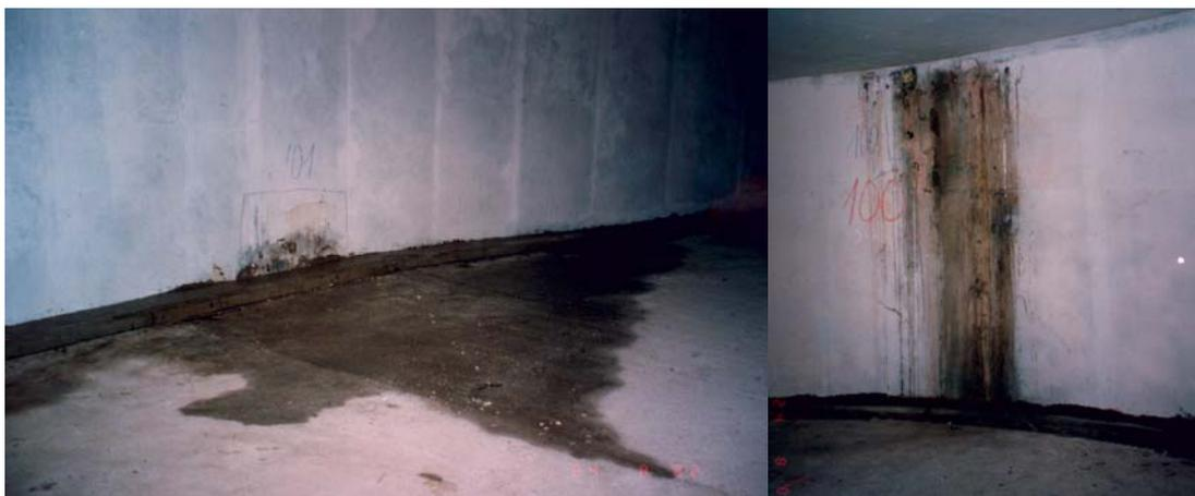
Fig. 2: Penetration of water through reinforced concrete walls of the underground garage.
