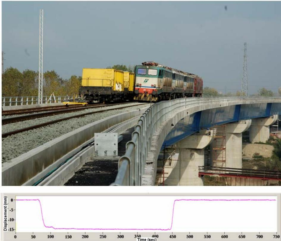
Figure 14: testing and radar image of the Indiano's bridge
