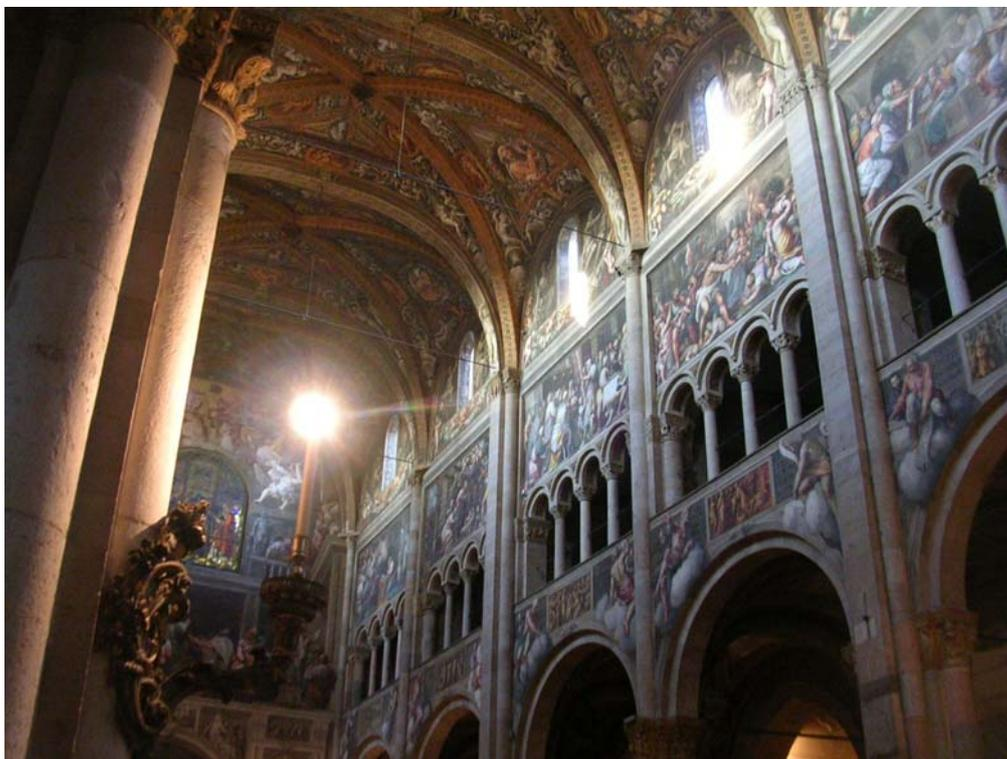
**Figure 2. The inside of the Duomo of Parma built from 1106. The roof vaults are visibly deformed. Paintings on the nave walls are by L. Gambara (1567-1571).**
