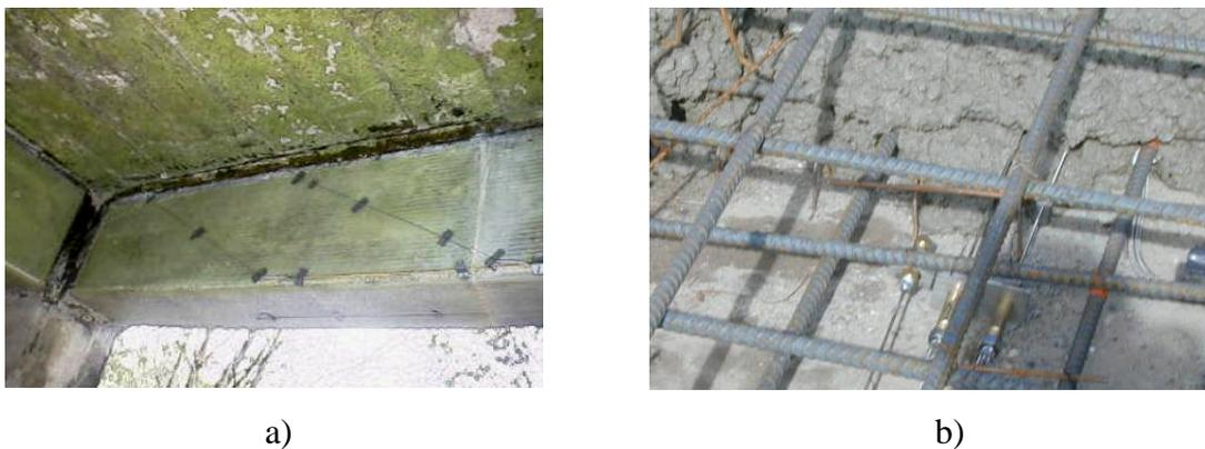
**Figure 6. a) Surface mounted fiber strain sensors on a bridge girder and, b) sensor embedment into a concrete slab prior to curing.**
