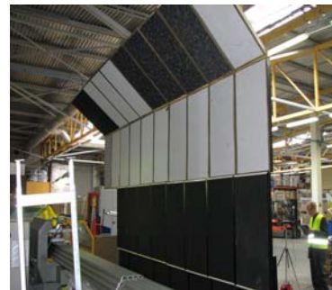
Fig. 6. General view of the acoustic partition wall in the workshop of aluminum pipe cutting
