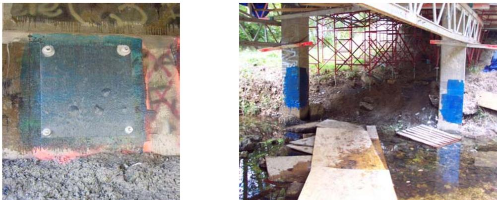
Figure 8. CFRP laminates with delaminations on south abutment and north bent
