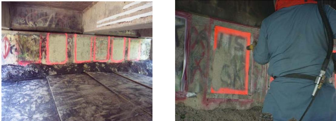
Figure 2. Surface Preparation on Abutment
