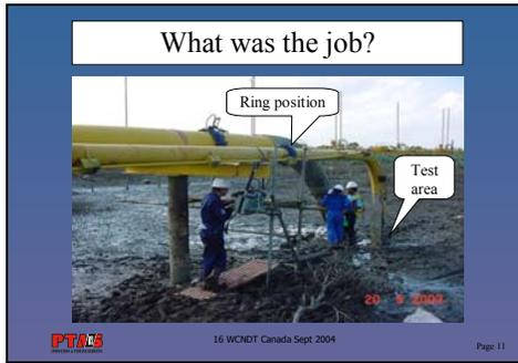
This slide is typical of the working conditions; this is in the tidal zone of a river estuary. For larger diameter pipes, an inflatable belt system is used. The system allows for a light flexible application of the technique to large diameter pipes. The normal range of inflatable rings is from 6 to 24 inches in diameter. (Larger pipes can be inspected, but on large pipes only large corrosion patches can be found.)
